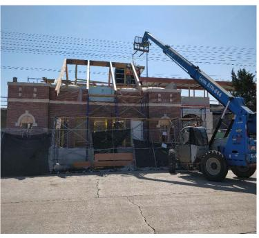
lighting, and electrical. The elevator shaft is completed and construction of the cab done inside of the elevator shaft. Finally, the main building is wrapping up with electrical, mechanical, lighting, and roofing elements in progress.
