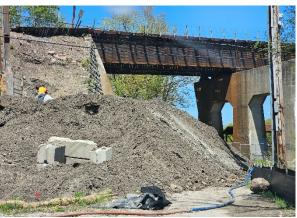
Workers removing loose material before installing earth retention system for the bridge.
