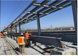
Installation of steel beams on station platform.
