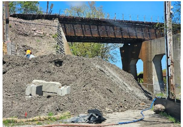
Workers removing loose material before installing earth retention system for the bridge.
