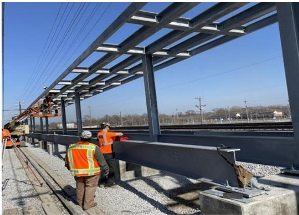
Installation of steel beams on station platform.
