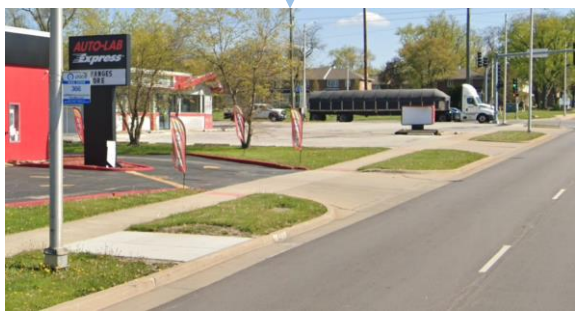
ROUTE 366 BUS STOP LOOKING SOUTH DOWN WESTERN AVENUE
