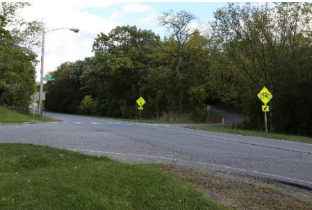
EXISTING 26 TH STREET CONNECTION TO THORN CREEK TRAIL
