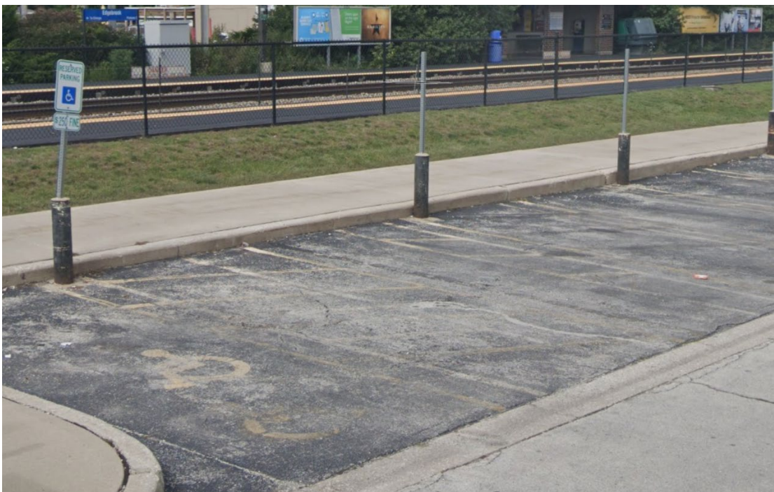
Image 2 (SE portion of Project Area): The ADA-parking stall painting is worn, ADA signs are missing, and blacktop pavement is buckling and unlevel. This access point lacks proper ADA tactile treatment.
