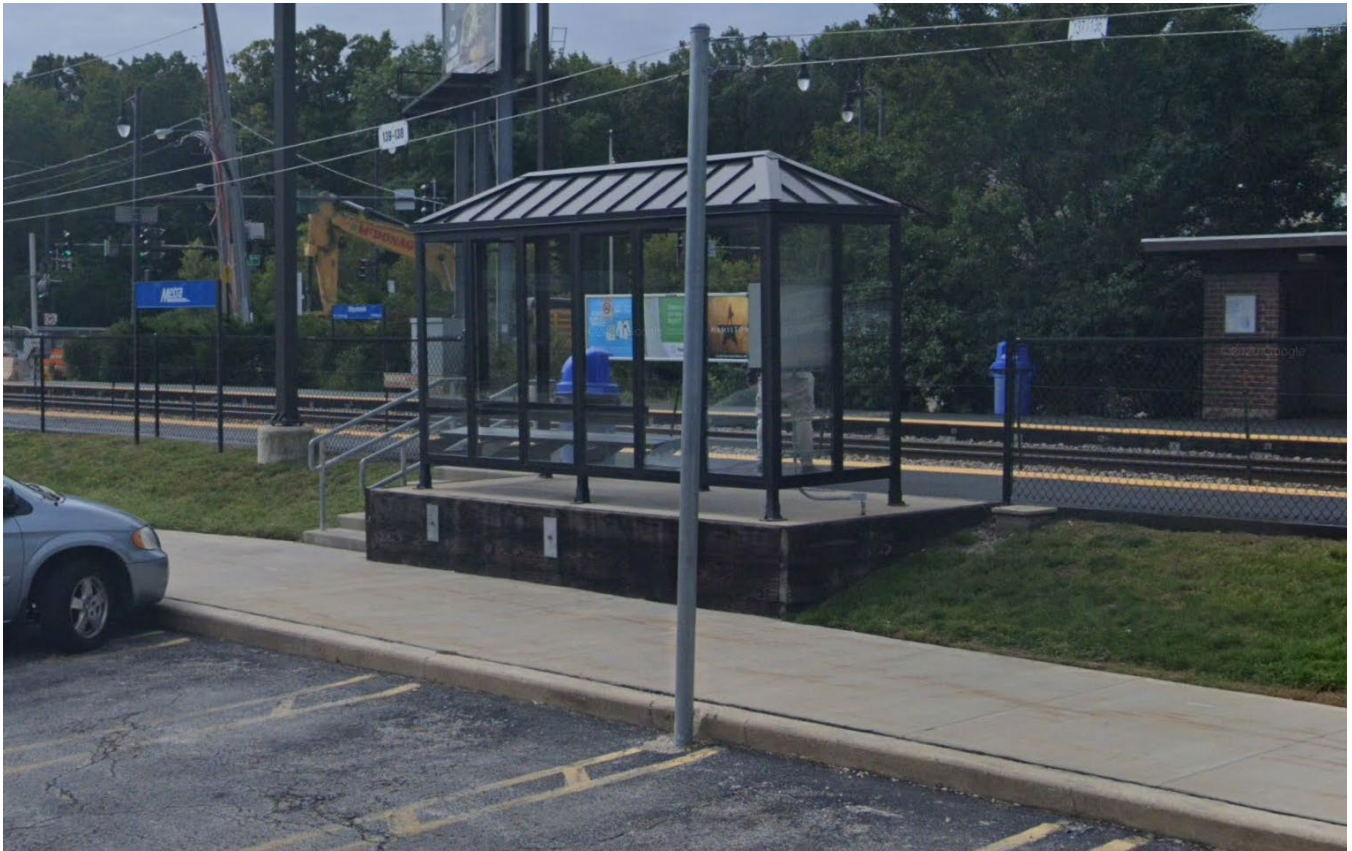
Image 3 (E portion of Project Area): The existing shelter fronting the eastern platform is small, not fully enclosed, lacks proper lighting, and does not provide adequate heating or climate-controlled space for passengers to keep comfortable during inclement weather.
