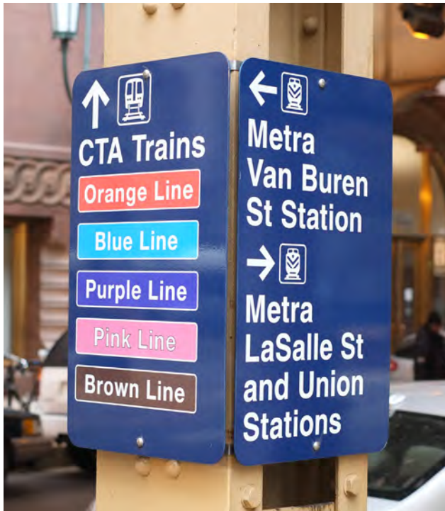
Two DSS-4 sign panels installed on a CTA elevated structure column with CMCC mounting brackets. Location: LaSalle Street
