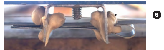
3 Photo Example of Epoxy Added to Bracket Scale: NTS
