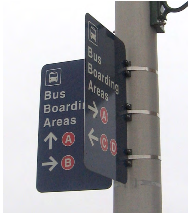
Two DSS-4 sign panels installed on a light pole with CMFS mounting brackets. Location: 95th and Western
