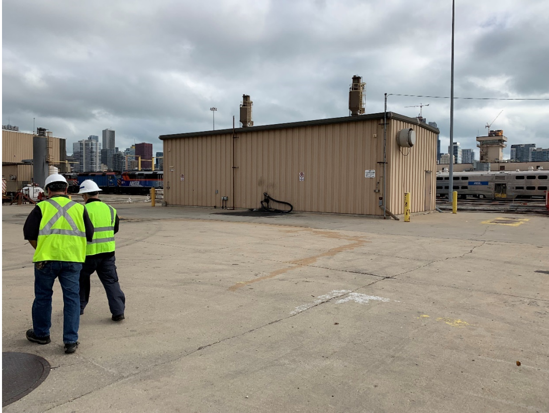
Figure 7 - 14th Street Shop Fuel Pumping Station
