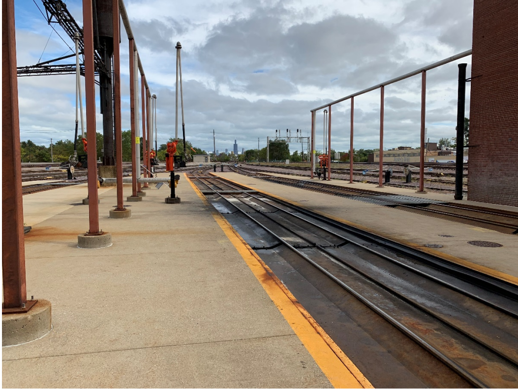
Figure 8 - M-19-A Exterior Fueling Rack
