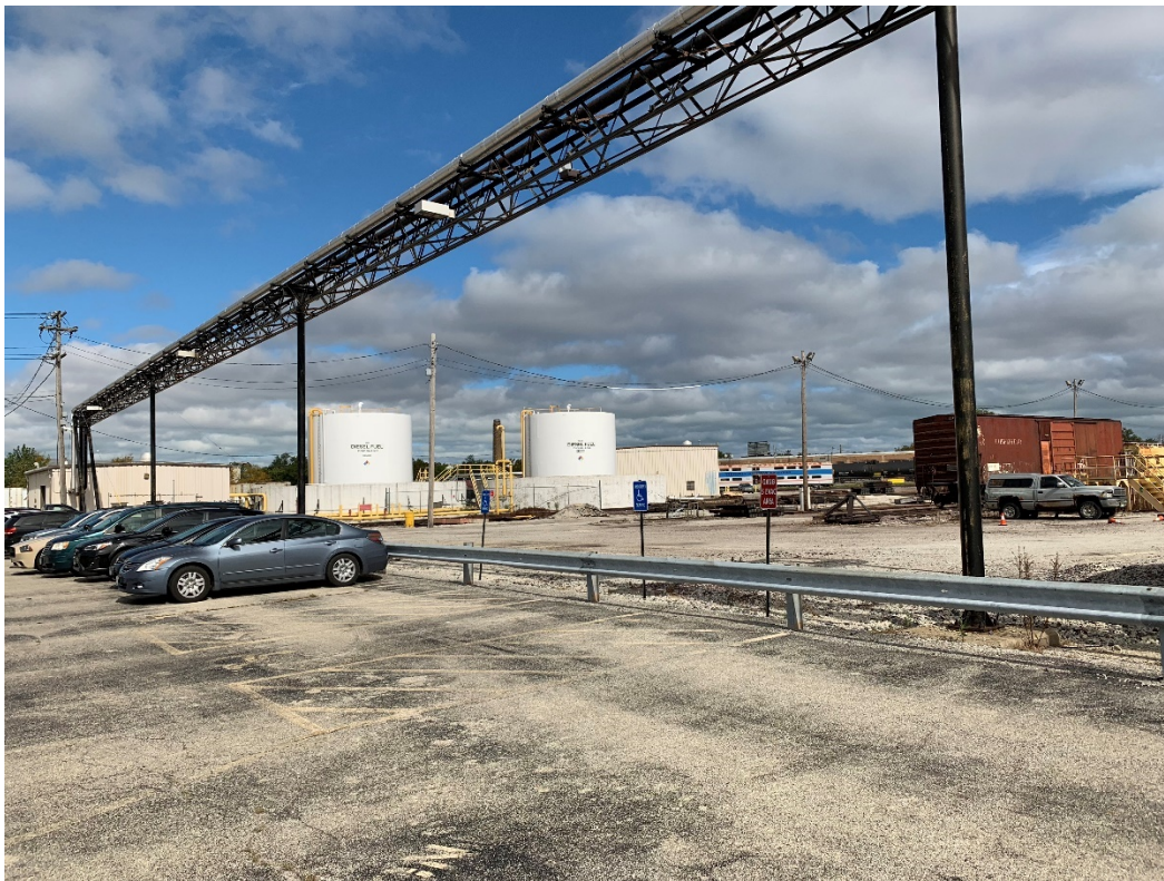
Figure 13 - M-19-A Fuel Pipeline Gantry, Pumping Station, and Above-Ground Tanks
