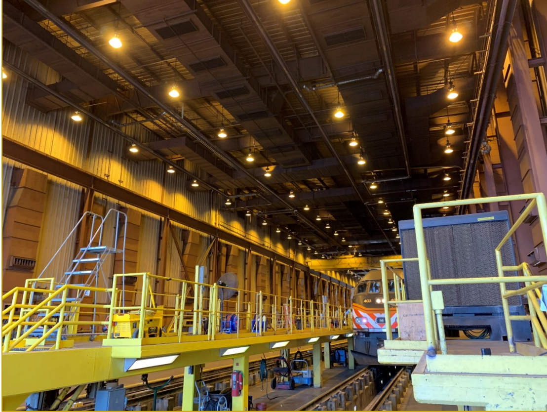
Figure 86 - Western Avenue Locomotive Shop Ceiling View
