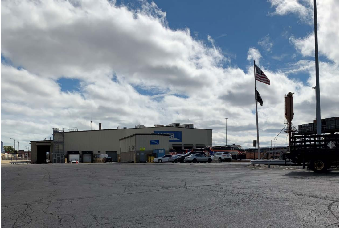
Figure 5 - Western Avenue Shop with Pumping Station in Foreground
