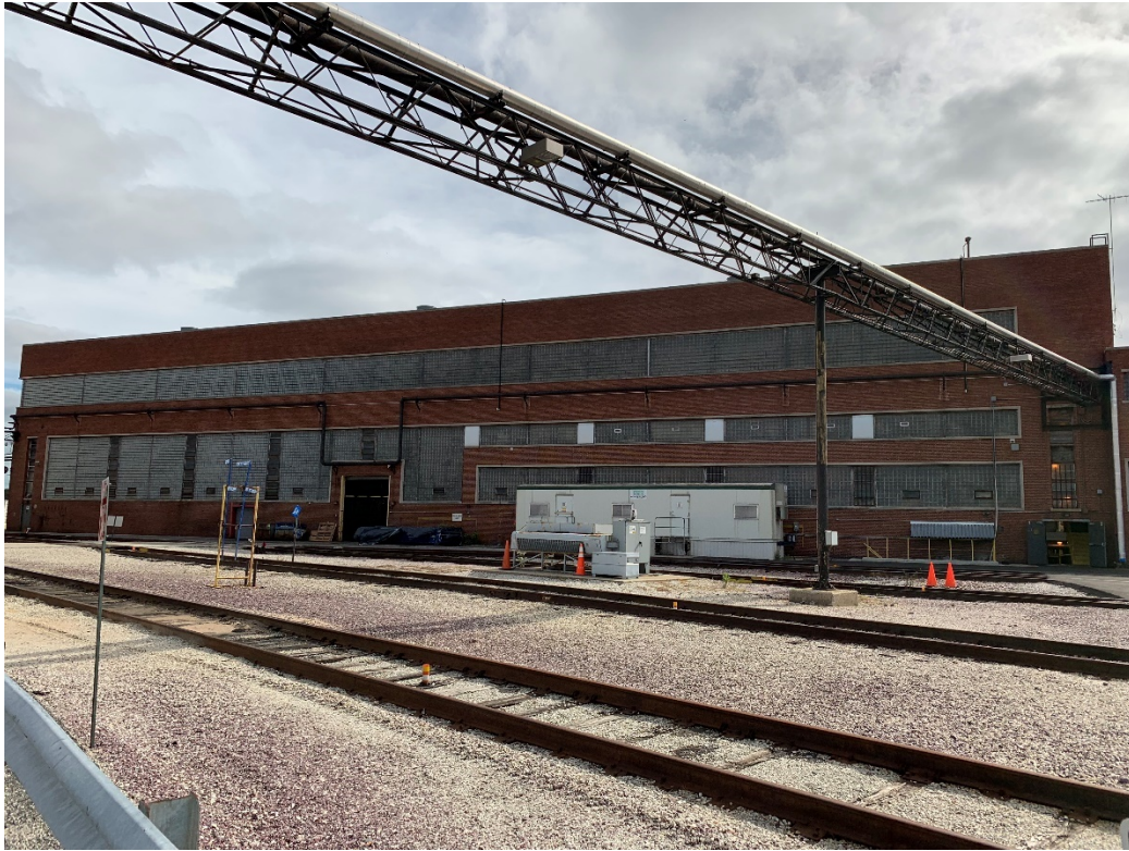
Figure 12- M-19-A Fuel Pipeline Gantry
