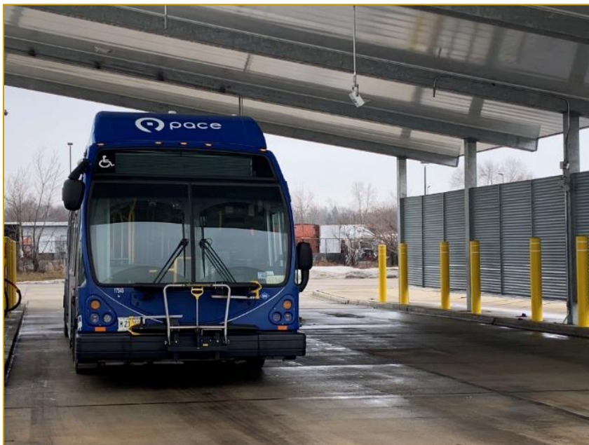
Figure 34 - Pace Bus within Fueling Shelter
