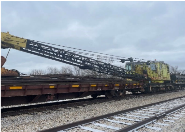
Existing Metra crane removing old ties from the right-of-way.
