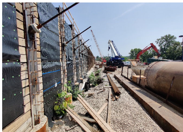
Workers doing final touches on retaining wall before concrete pours.
