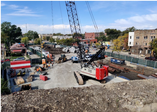
Crane on site to transfer sheet piles to be driven for the earth retention system on the new Auburn Park Station.
