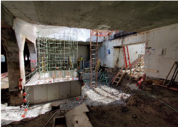
Construction of the elevator shaft at 79 th Street Station.
