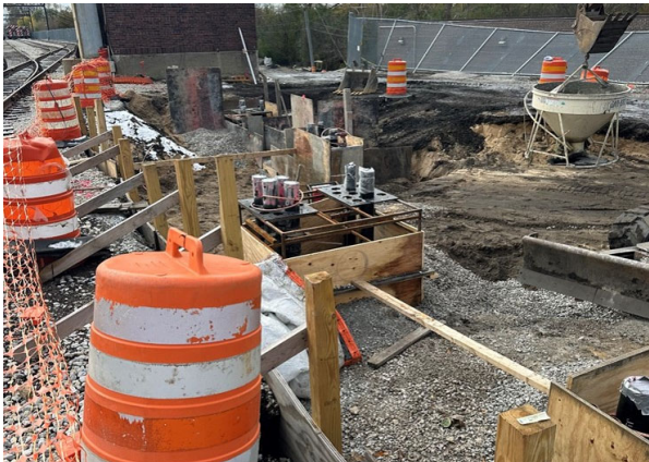
Duct bank concrete pour for Matteson Substation.
