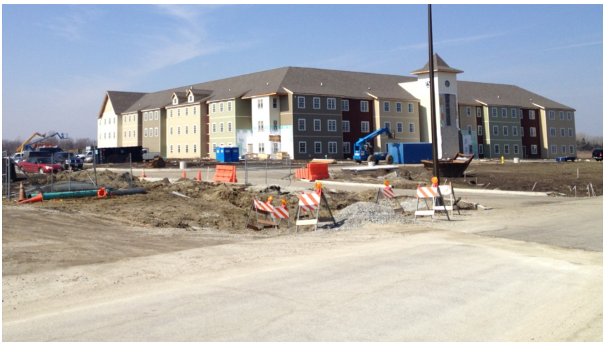
Student Housing under construction. (Photo Credit: RTA)
