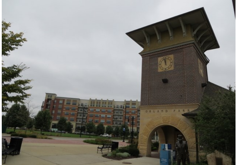
143rd Street Metra Station and Ninety 7 Fifty on the Park (Photo Credit: RTA)
