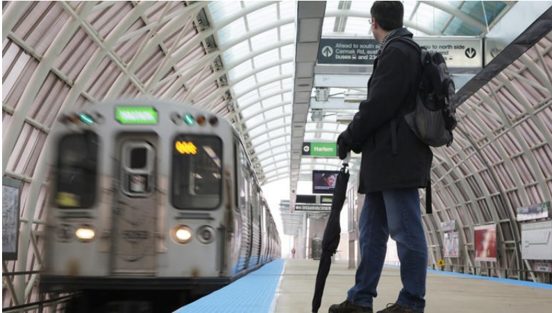
The new Cermak-McCormick Place Green Line Station.
