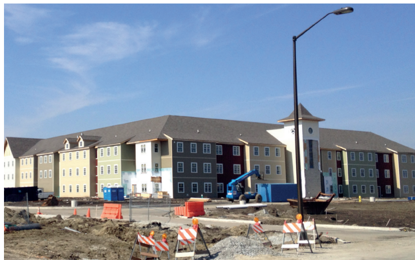
Governor's State student housing under construction
