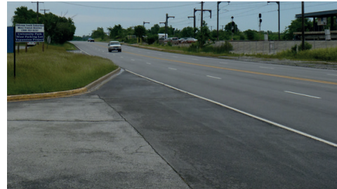
Governors Hwy near the University Park Metra Station
