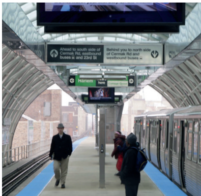
The new Cermak-McCormick Place Green Line Station (Photo Credit: Stacey Wescott, Chicago Tribune)
